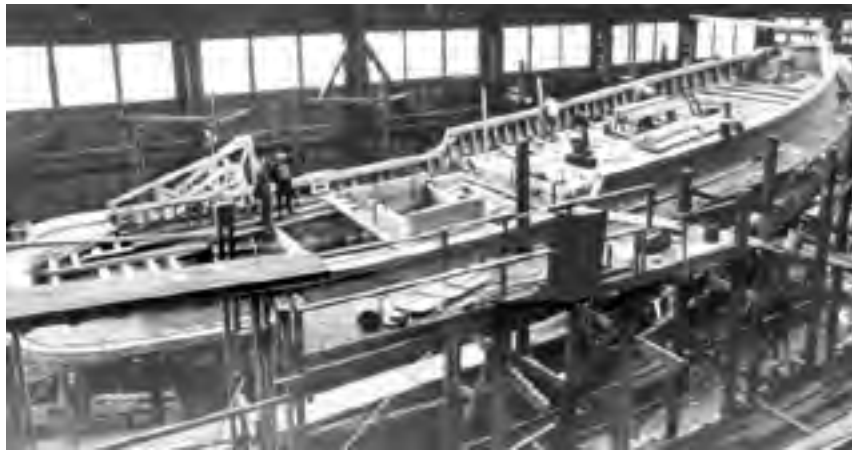
Building the John N. Cobb, NOAA
